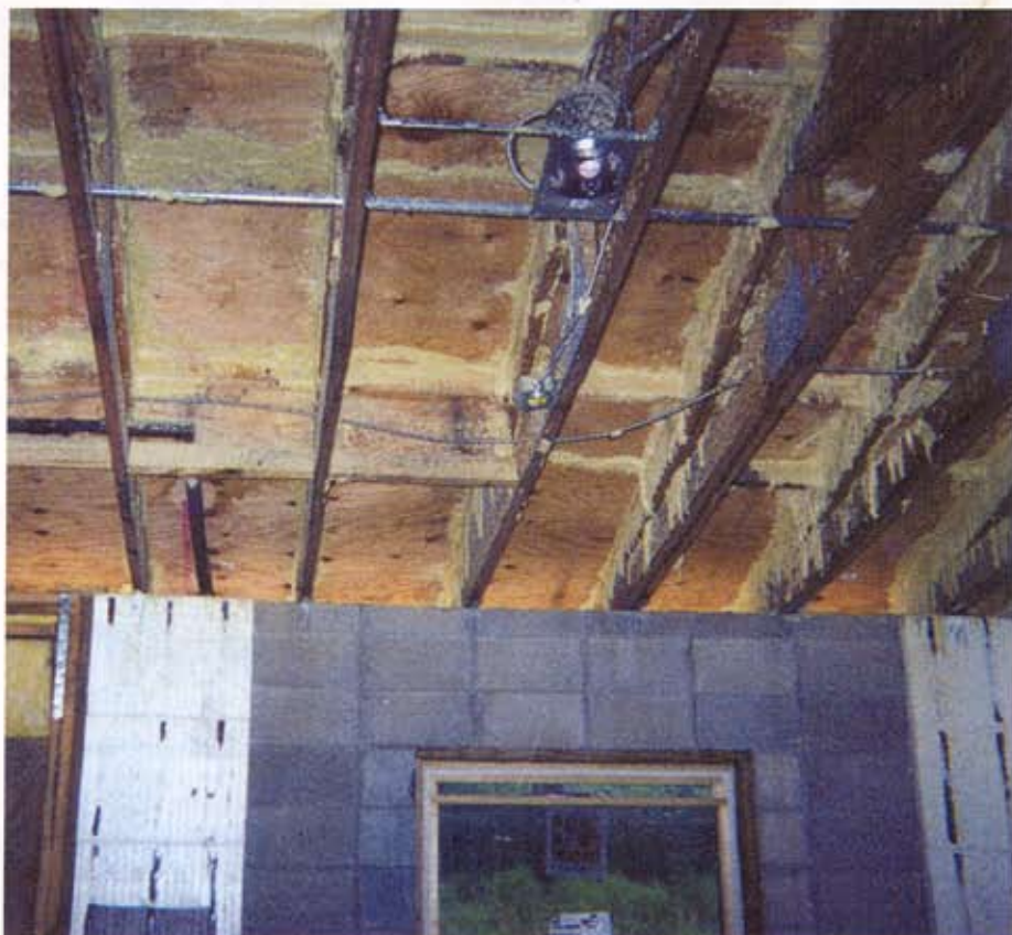
Working in conjunction with the University of Florida's Shimberg Center for Affordable Housing, several Florida spray foam contractors have contributed their time and materials to the building of Windstorm Damage Mitigation Training and Demonstration Centers, also known as Hurricane Homes (bottom left, page 24). In an effort to increase a structure's wind and water resistance, SPF adhesive is spray-applied to the roof sheathing of these demo homes (above and below).
