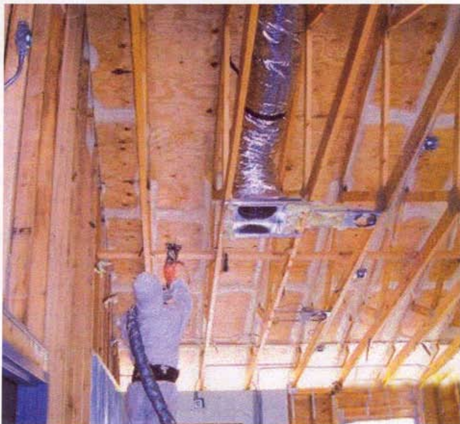
Working in conjunction with the University of Florida's Shimberg Center for Affordable Housing, several Florida spray foam contractors have contributed their time and materials to the building of Windstorm Damage Mitigation Training and Demonstration Centers, also known as Hurricane Homes (bottom left, page 24). In an effort to increase a structure's wind and water resistance, SPF adhesive is spray-applied to the roof sheathing of these demo homes (above and below).
